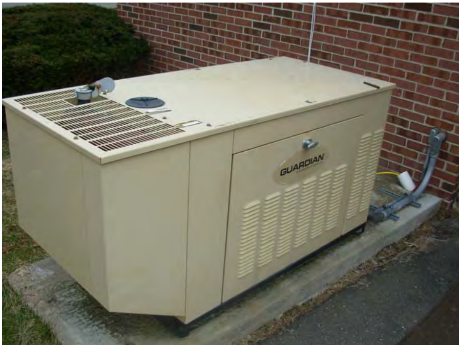
11. Emergency generator serving Cmnty. Bldg.
