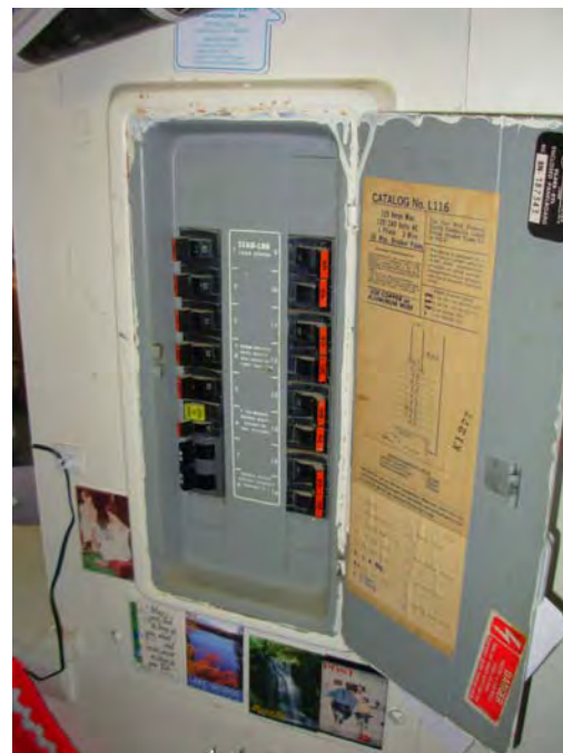
16. Federal Pacific Stablok circuit breaker panels to replace
