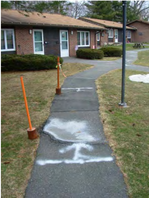
1. Sidewalk sections to be re-paved, trip hazards
