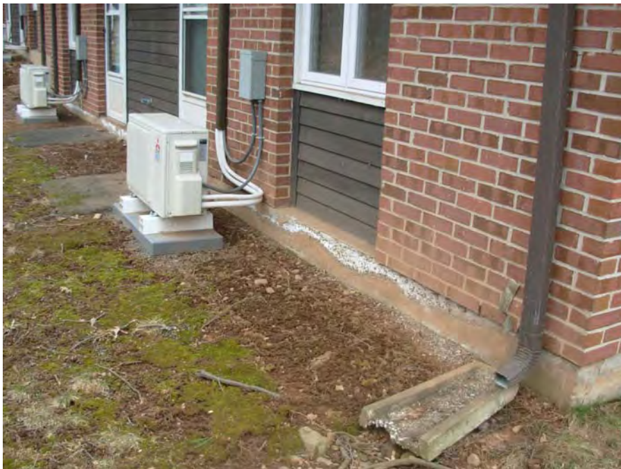
3. Spalling foundation at rear of Units 21, 22, 23
