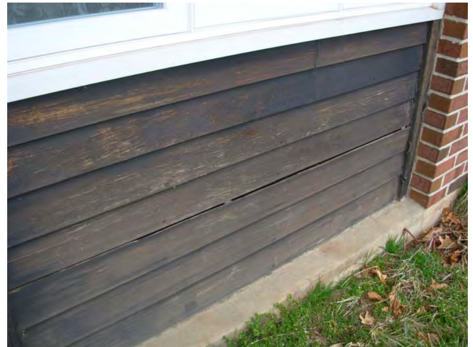
4. Wood siding damage and deterioration
