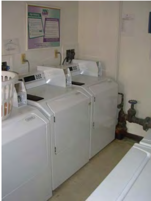
9. Laundry facility equipment spacing too narrow
