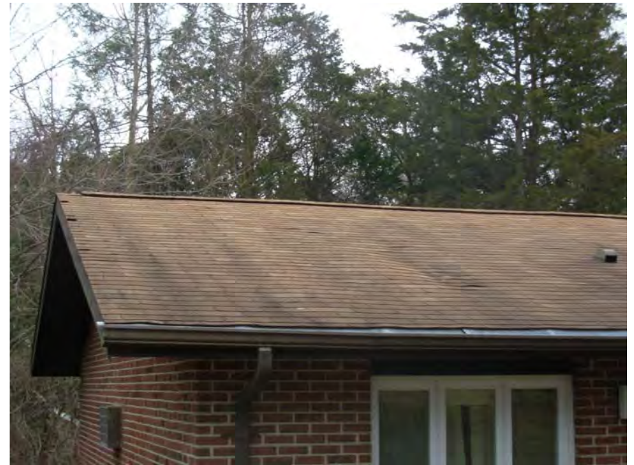
6. Lifting and stained shingles, decking deflection
