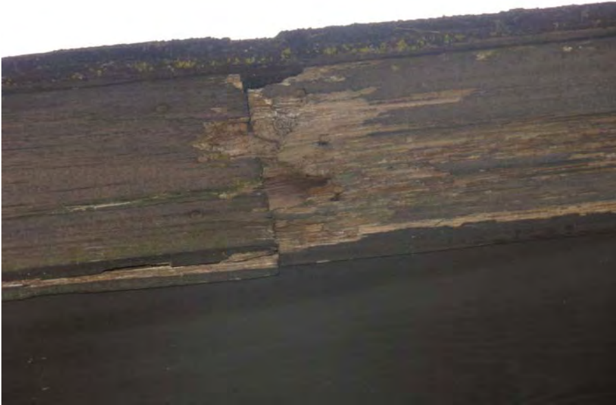
5. Wood trim deterioration
